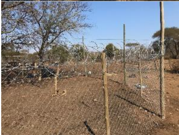
A boma before (top) and after (bottom) reconstruction. The rickety fence of the original boma no longer acted as a barrier to either cattle or wildlife and was replaced with a sturdy 2m high fence capped with razor wire for extra protection
